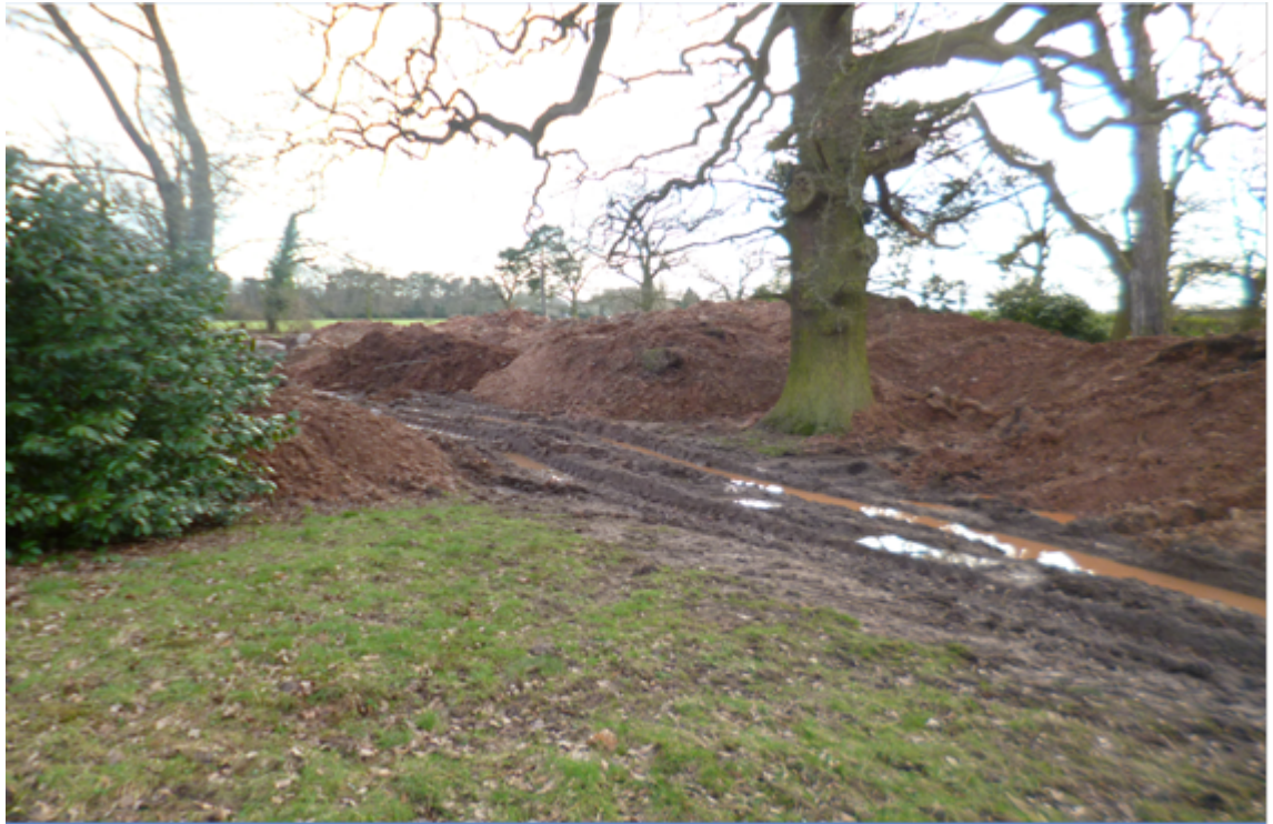
Damaged soil structure from the passing site vehicles within the Root Protection
